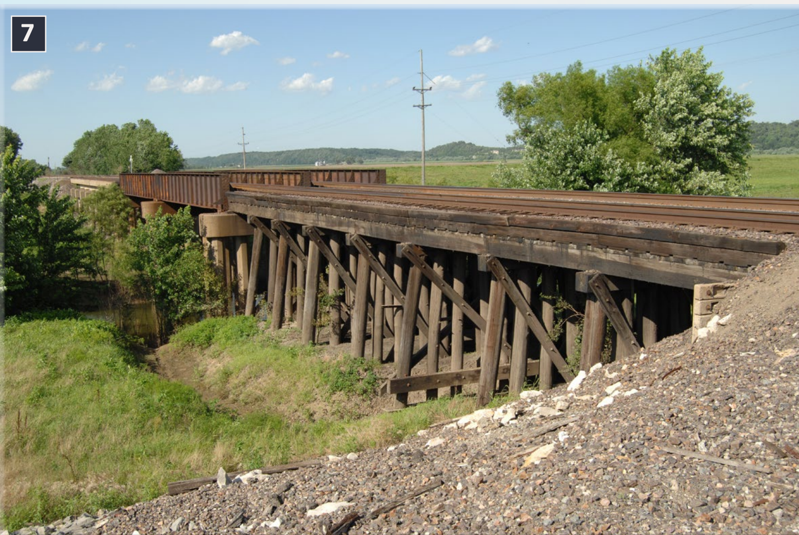
7. The wooden trestle supporting the approach span contrasts with modern segmental concrete work supporting the steel through-deck bridge. Dirk Reynolds photo.
