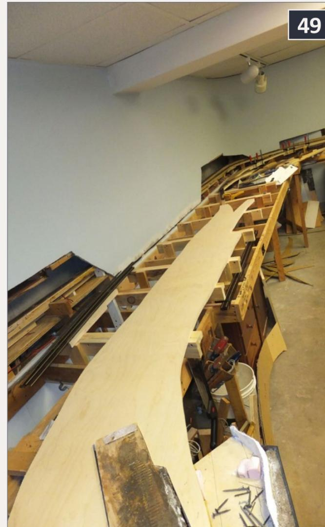
49: Once I'd arrived at a track layout, I used the track arrangement to mark the cuts on the big sheet of plywood, and the here is the result. Note the cut at the bottom to fit existing sub-roadbed.
