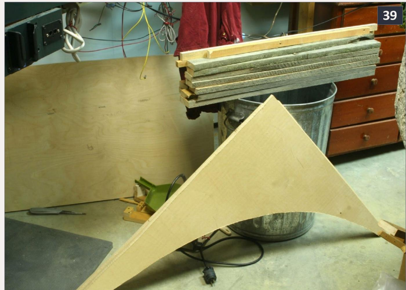
**39:** One of the plywood corner formers used to create the curved corner. The vertical pieces that would act as studs are stacked on top of the garbage can, ready to assemble and install.
